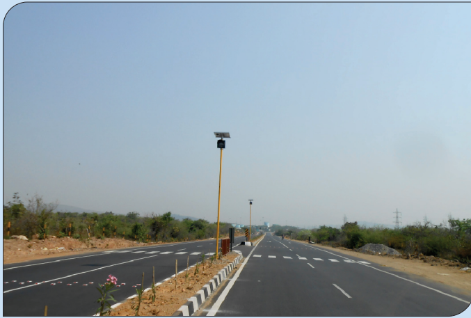
HKR Roadways Limited
